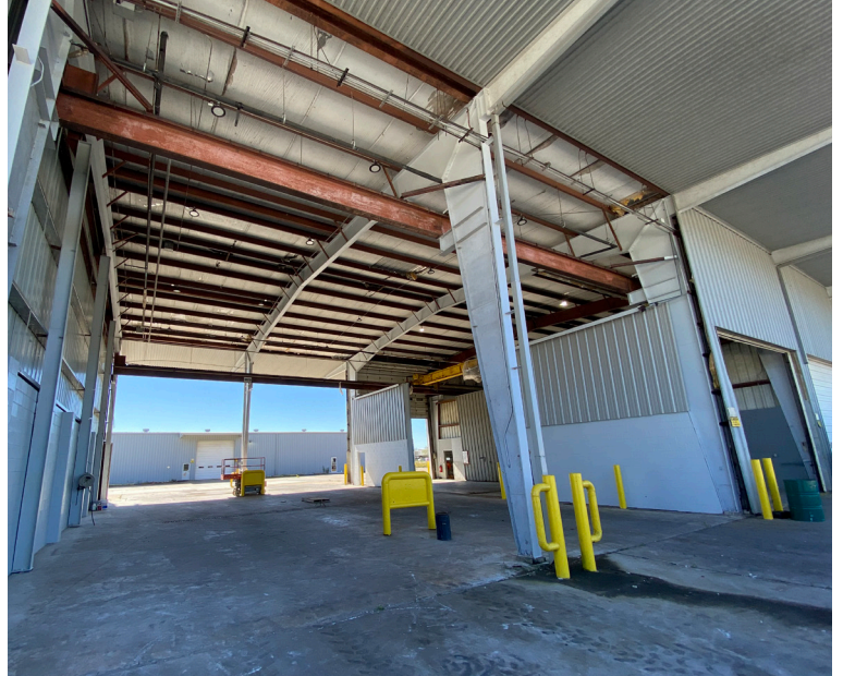
WAREHOUSE A - TRUCK WASH BAYS
