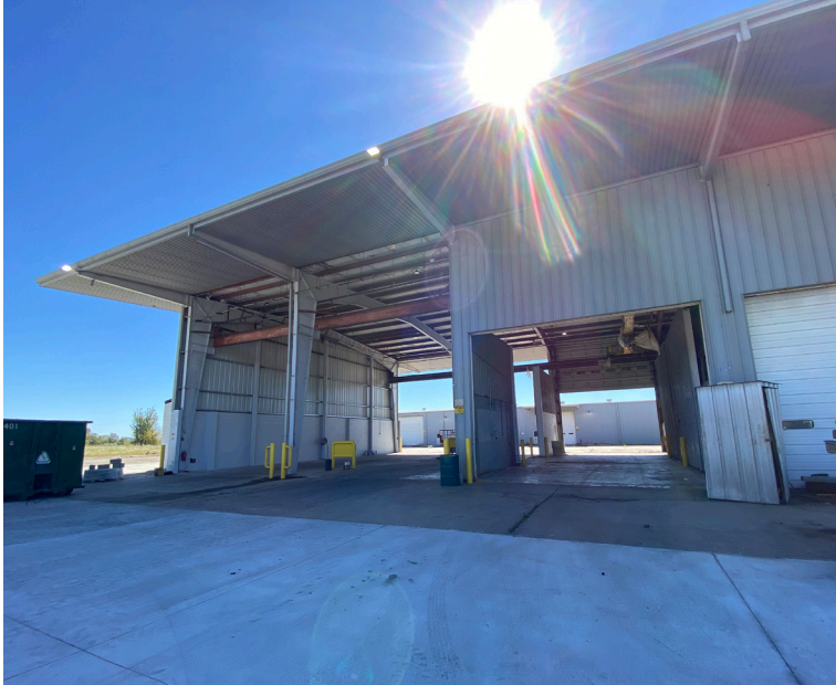
WAREHOUSE A - DRIVE-THROUGH
