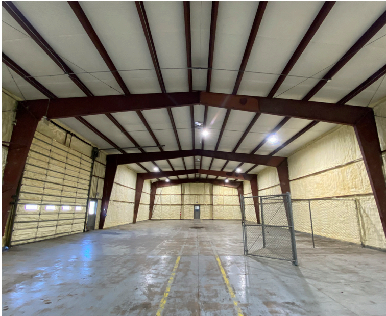
WAREHOUSE B - WAREHOUSE INTERIOR
